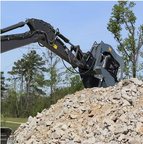
Stand the excavator on top of the material and load the loose material into the screener. Be careful of metallic material, as it may become trapped in and damage the meshes.
