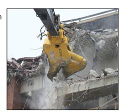
Whether a GRX, linkage tool or GDT, Genesis concrete processors spend most of their lives in extremely abrasive environments and require regular service intervals. Hard-surfacing is a common method for protecting surfaces and reducing component and structural wear. Hard-surfacing patterns and application instructions can be found in the product <u>Safety & Operator's Manuals</u>.
